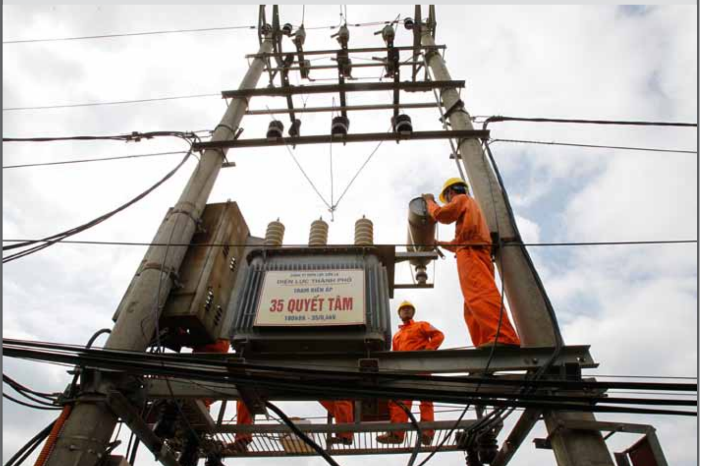
Workers repair an electric transformer in Son La province, Vietnam. REUTERS/Kham
